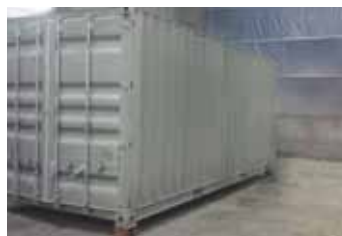
Application of fast cure Interzinc 22 and tie coat/intermediate coat on day 1
