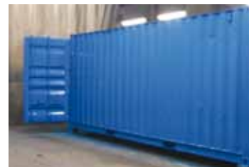
Application of Interthane 990 finish coat completed on day 2
